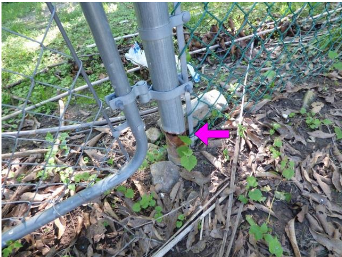
13.0 Picture 9 - Gate post rusted through
