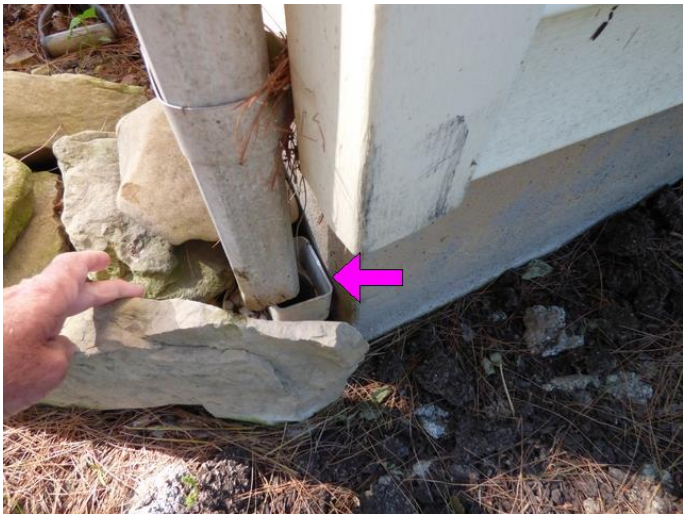
13.0 Picture 7 - Downspout disconnected
