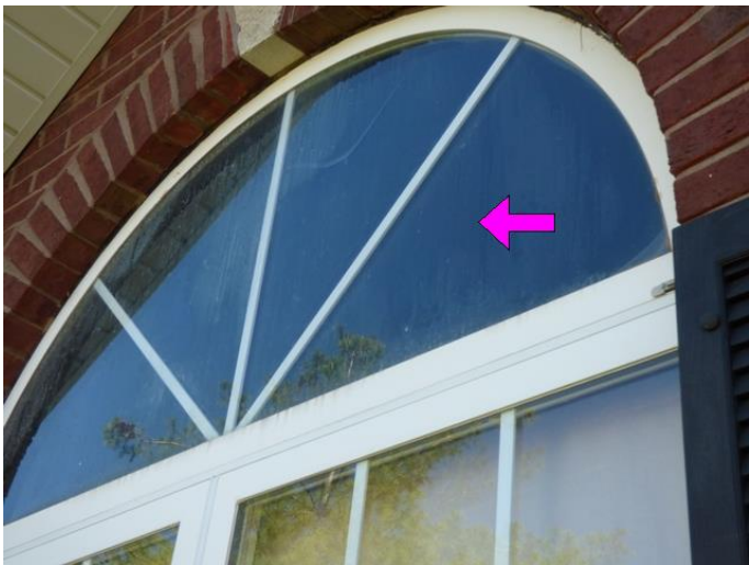
13.0 Picture 3 - Thermal seal broke
