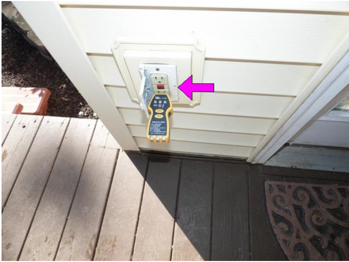
13.0 Picture 5 - Exterior GFCI outlet defective
