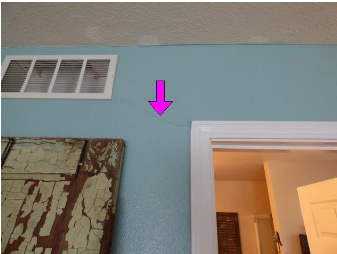
13.0 Picture 19 - Wall crack
