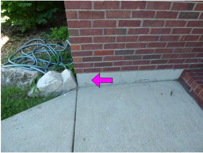
13.0 Picture 1 - Foundation corner crack
