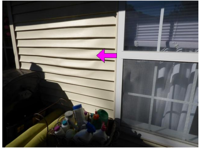
13.0 Picture 6 - Heat warped from BBQ grill
