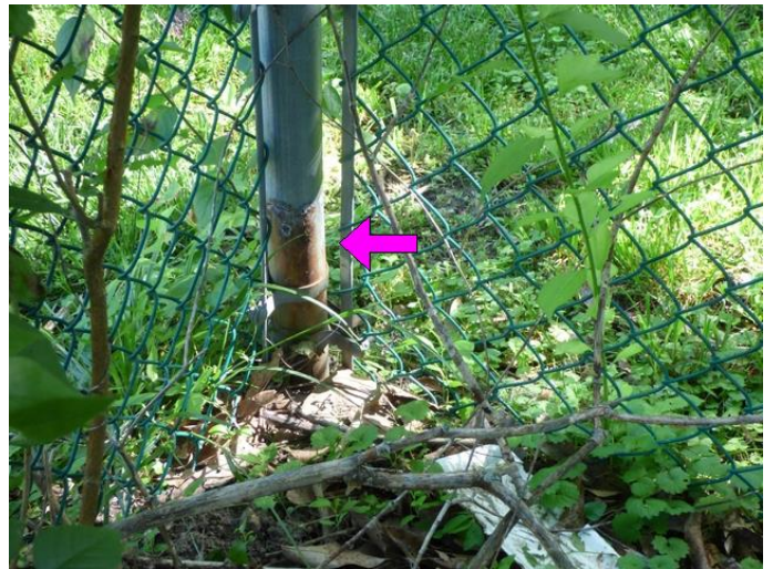
13.0 Picture 10 - Corner post rusted through
