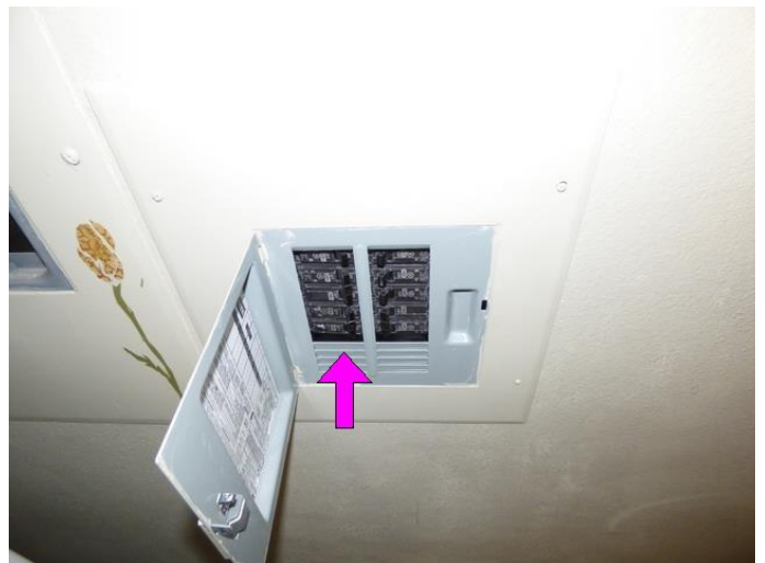
13.0 Picture 16 - Subpanel not flush with wall
