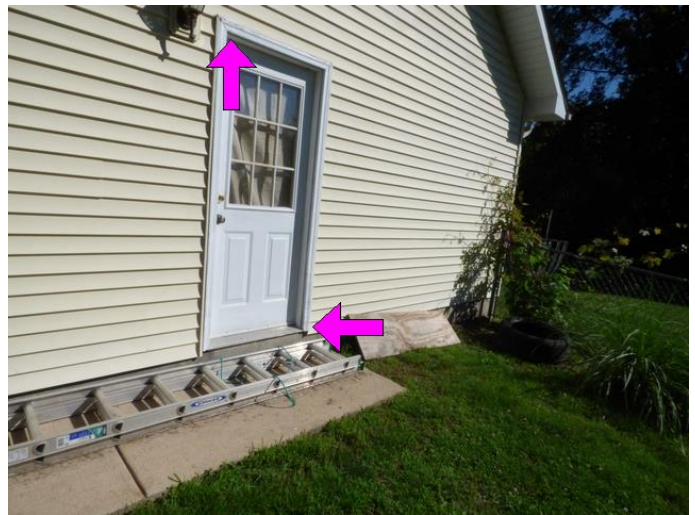
13.0 Picture 4 - The door jamb/trim has moisture damage
