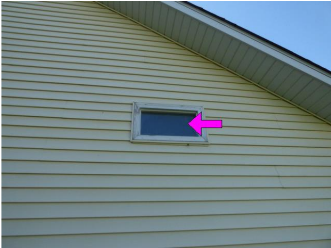
13.0 Picture 11 - Thermal seal broke
